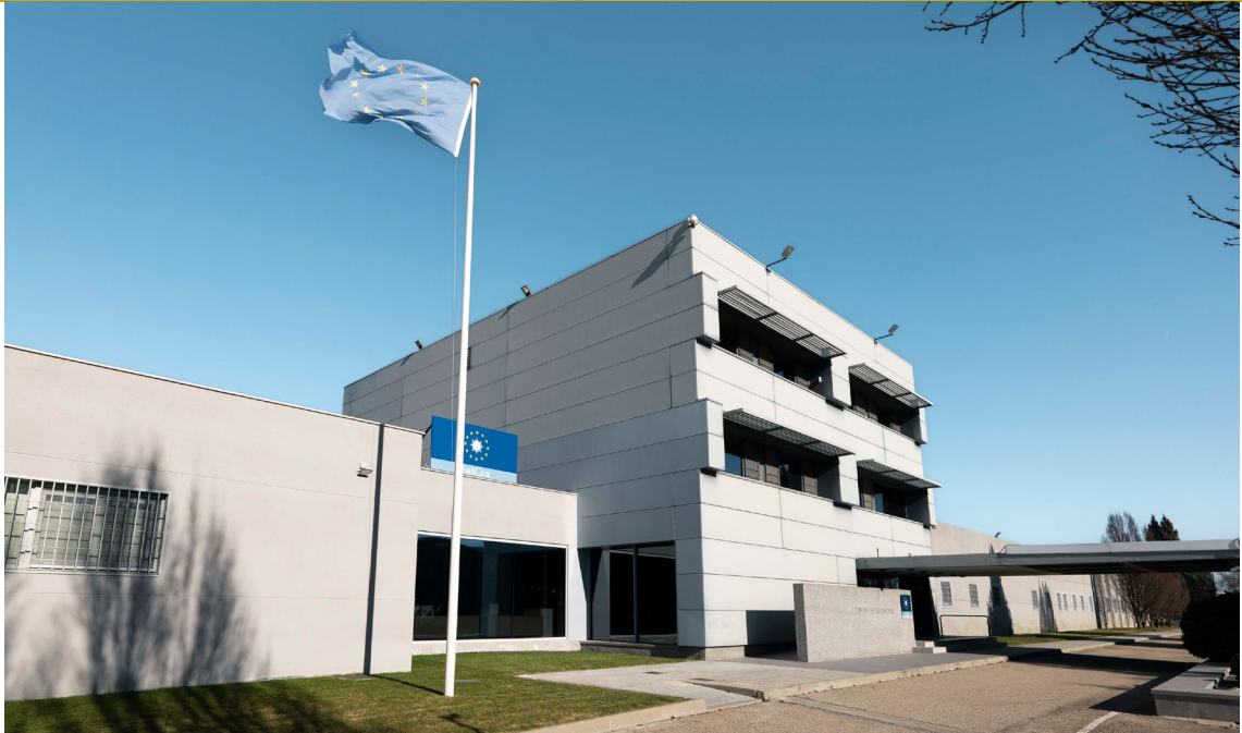
Overview of new SatCen building extension
